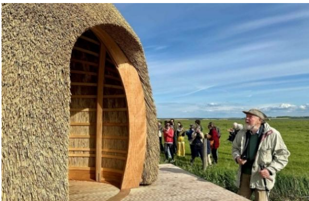
Figure 32. Bird watching Shelter made from local reed and local elder tree, Baltic Sea / Germany
