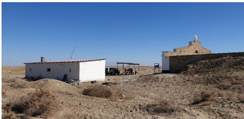
Backside of the Fish Processing Factory with picnic shelter in front and ranger house (view to Sudochye Lake)
